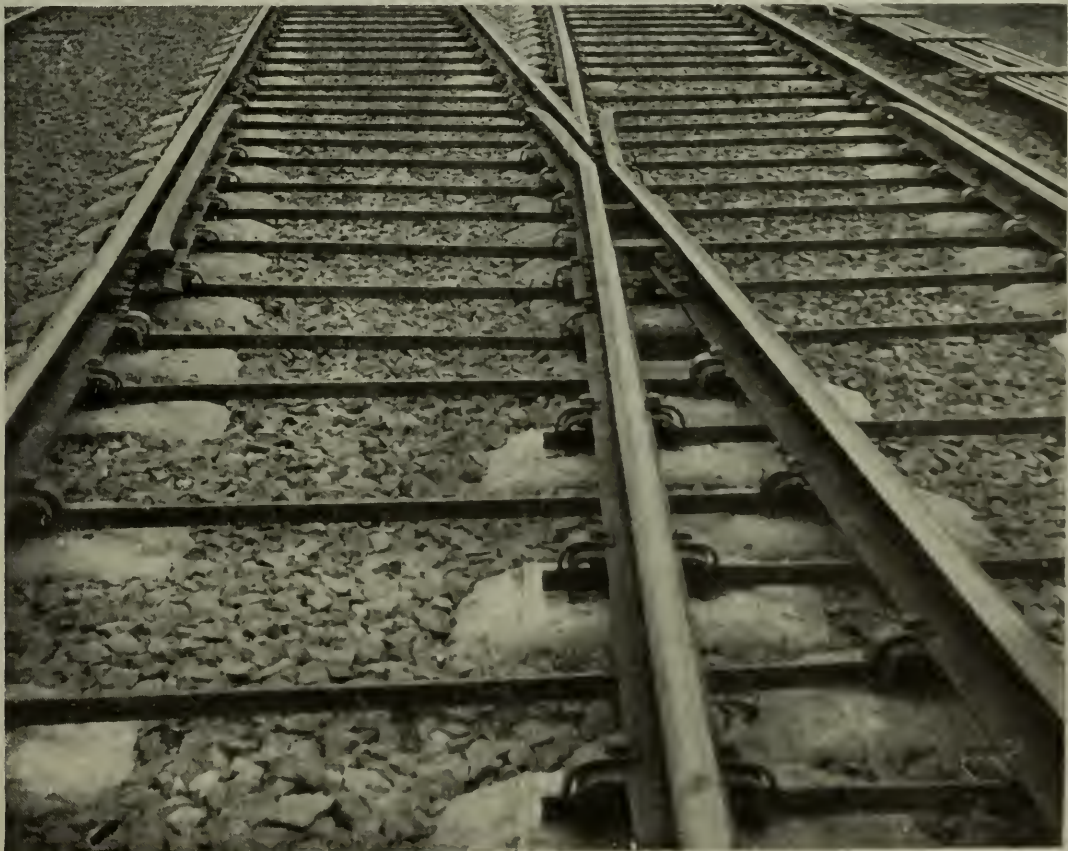
GREEN-MOORE REINFORCED CONCRETE SLEEPERS.
